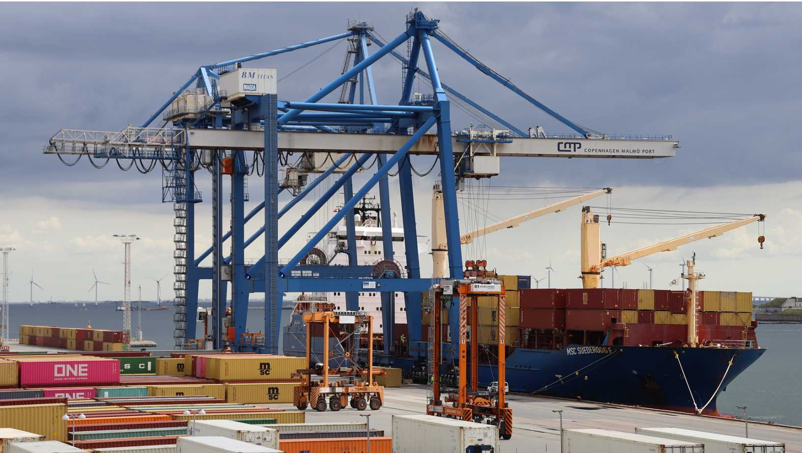
CMP's container terminal in Copenhagen
